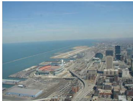
Cleveland Lakefront with Confined Disposal Facilities (CDFs) adjacent to Burke Airport
